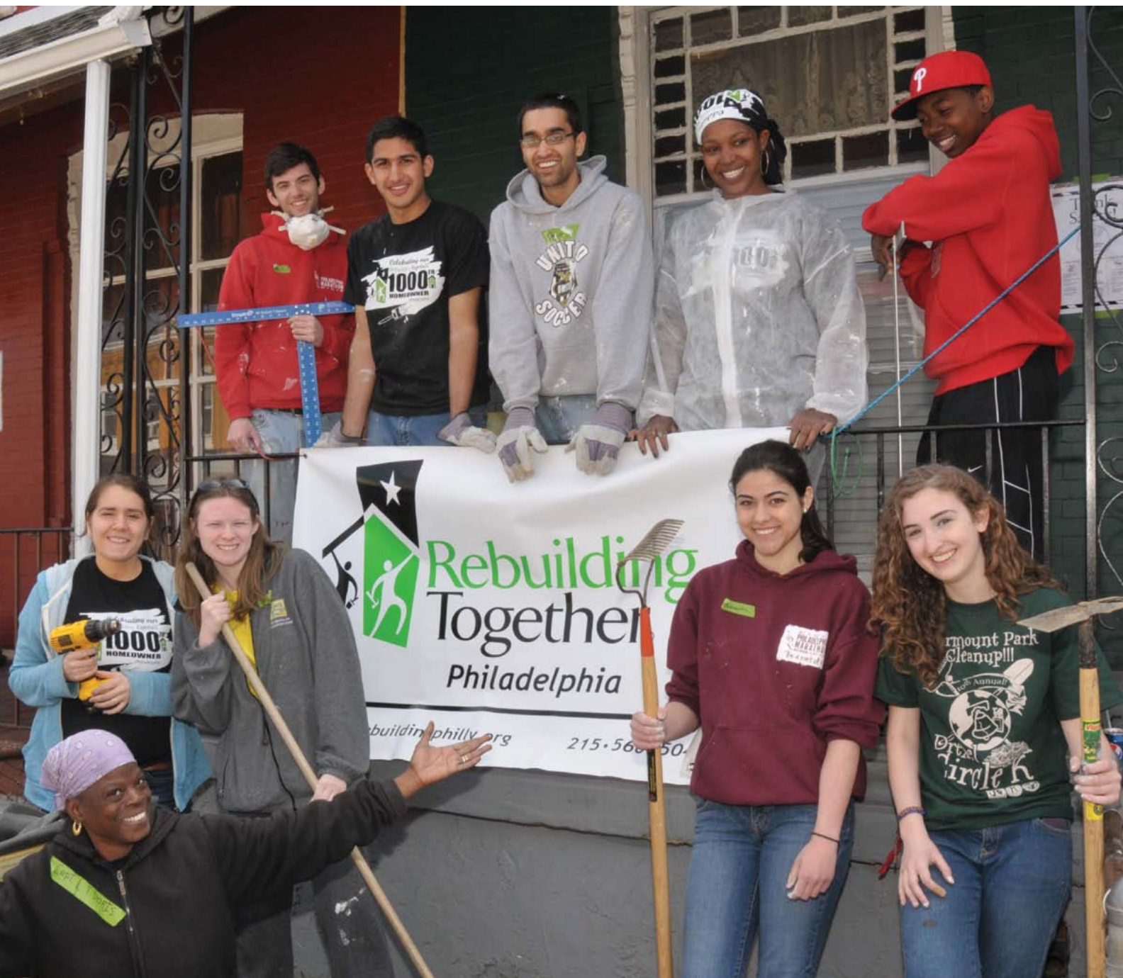
Drexel students on Alternative Spring Break rebuild a neighborhood block alongside community members.
