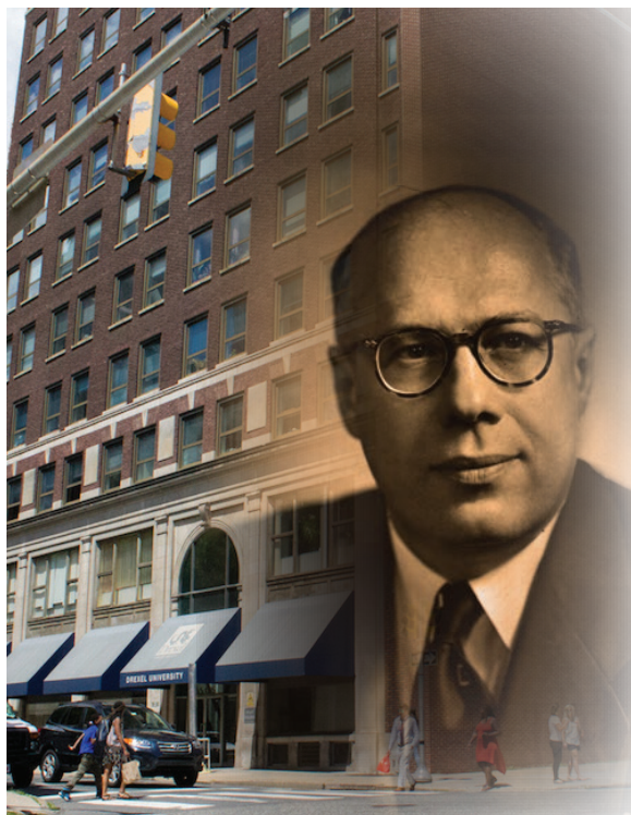
Purchased by Hahnemann Medical College in 1972, the Schaff (now Bellet) Building lost its easternmost portion to eminent domain in 1974 to accommodate the widening of 15th Street.
