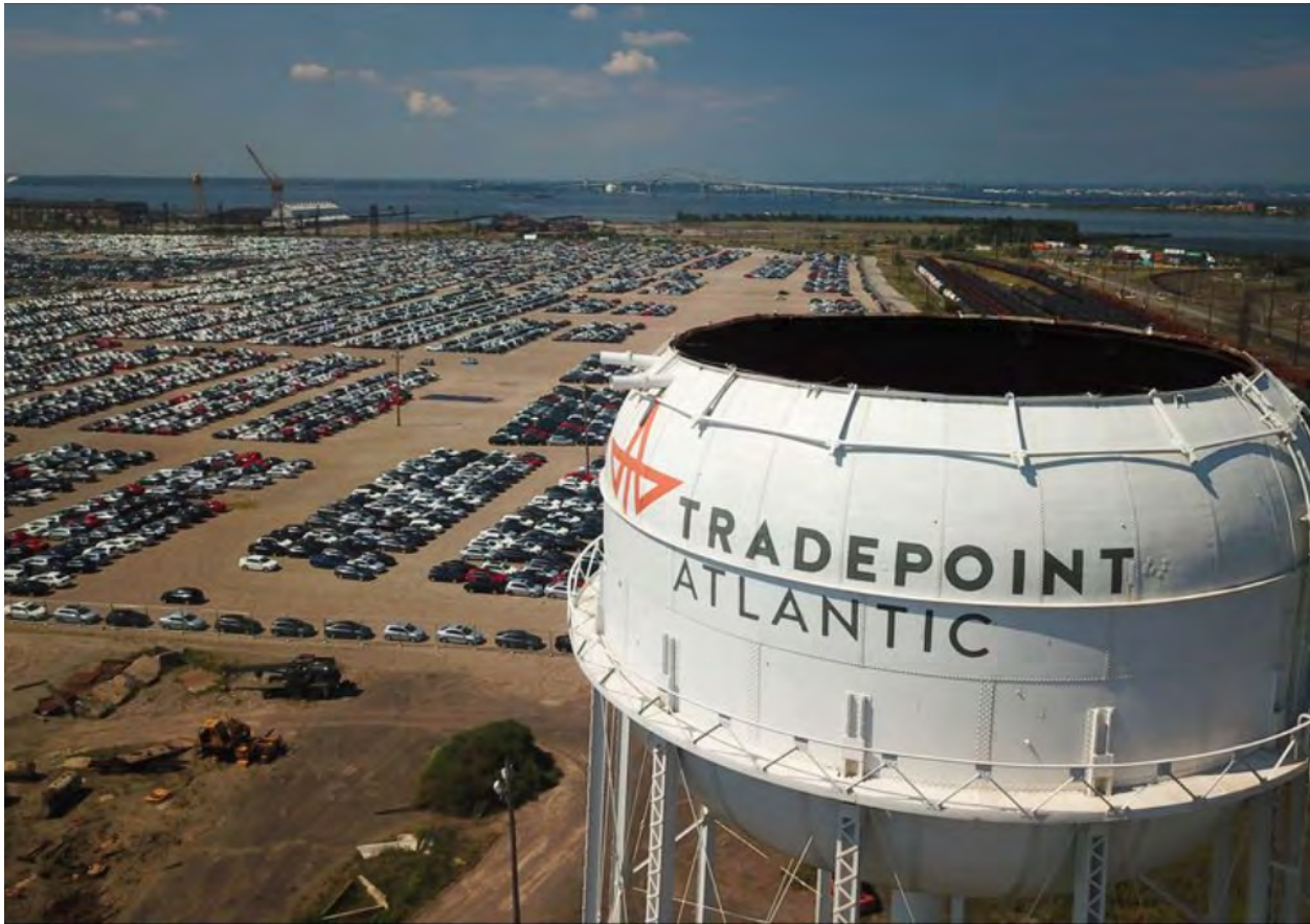
Industrial reuse followed remediation at Hilco's Tradepoint Atlantic site. Photo credit: Hilco Redevelopment Partners.
