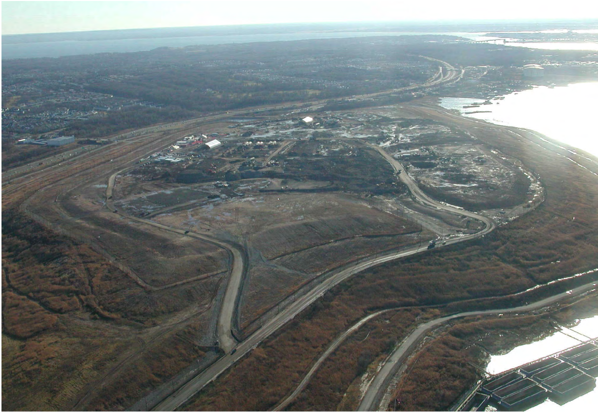
Aerial view of Freshkills Park under construction.
