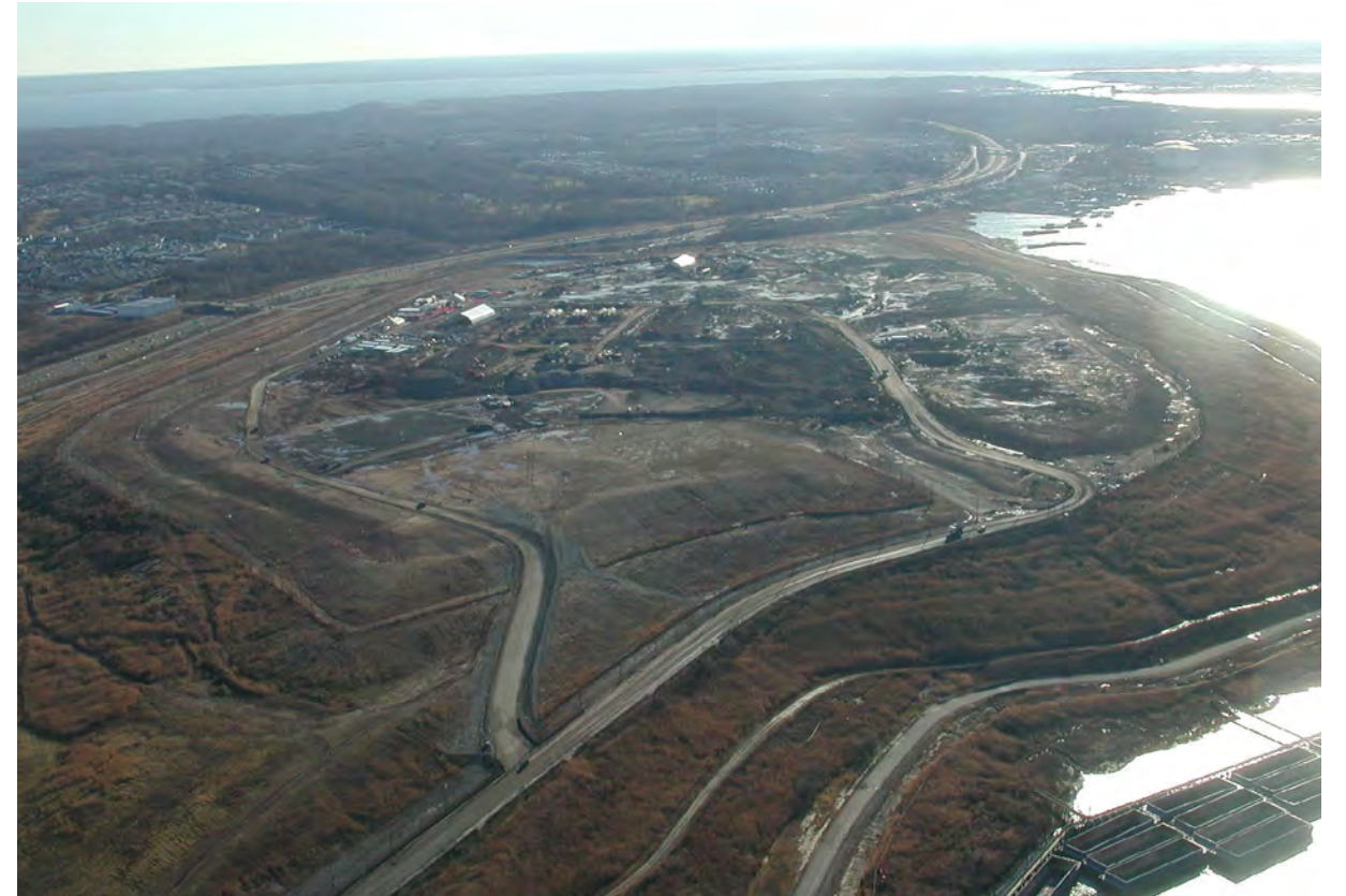
Aerial view of Freshkills Park under construction.
