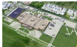
OKCWorks - multi-tenant business campus, 2 million sq. ft
