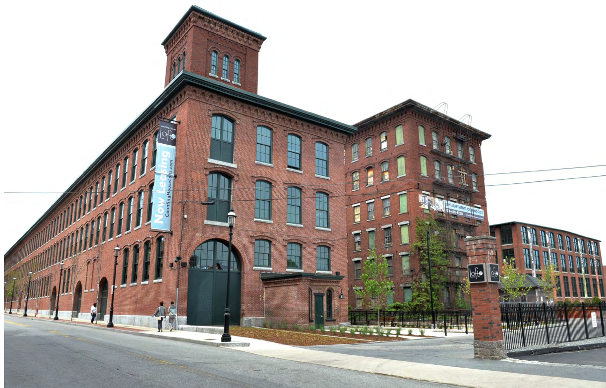
Figure 08: Examples of adaptive reuse in Lowell, MA. The Counting House (left) is a converted mill that houses a 52-unit mixed-income development with commercial space, with the 170-year-old Adden Building (middle) and Loft Two Seven (right), also comprised of mixed-income units. These developments are part of the Hamilton Canal Innovation District, another redeveloping former-industrial historic district adjacent to downtown Lowell.
