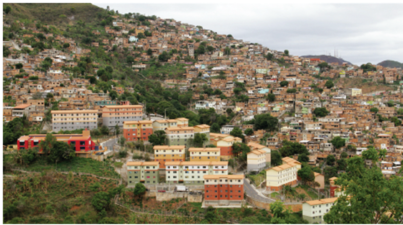
Figure 1. Vila Viva Project in Aglomerado da Serra, Belo Horizonte. Source: URBEL/PBH. Available at: http://www.Flickr.com/photos/portalphb . Public domain. undefined
