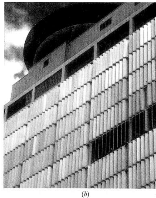
Fig. 6.17 (a) Movable fins. (b) Movable fins are positioned according to the sun's position at the Ala Moana office building in Honolulu, Hawaii. These effective shading devices were removed when the building was remodeled to make it look more contemporary. (Drawing by Erik Winter, photo by Alison Kwok; © 2004 Alison Kwok; all rights reserved.)
