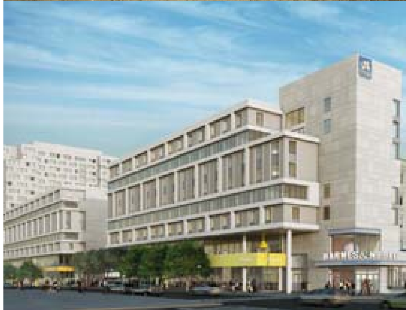
The ground-breaking ceremony and initial renderings for Chestnut Square. Through a partnership with American Campus Communities, Drexel will add 861 beds to its campus when this project is completed in Fall 2013.
