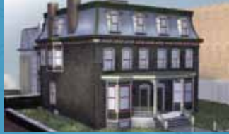
DREXEL SMART HOUSE Renovation in progress.
