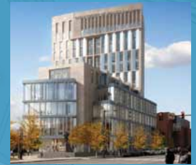
LEBOW COLLEGE OF BUSINESS BUILDING Opening Fall 2013.
