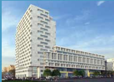
CHESTNUT SQUARE Student housing/retail at Creese Student Center and MacAlister Hall; opening Fall 2013.
