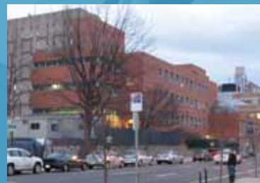
STRATTON HALL RENOVATIONS Design in progress.
