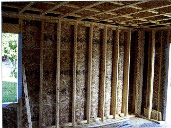
Double walls before (left) and after (right) the cellulose insulation was installed.
