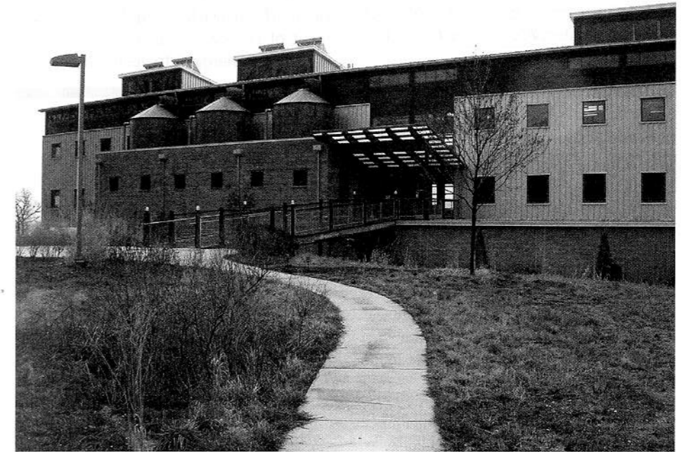
Fig. 2.13 North (inland) façade of the Philip Merrill Environmental Center showing the visual impact of rainwater collection intent and solution. Water conservation has informed this façade. (Photo © 2004 Walter Grondzik; all rights reserved.)
